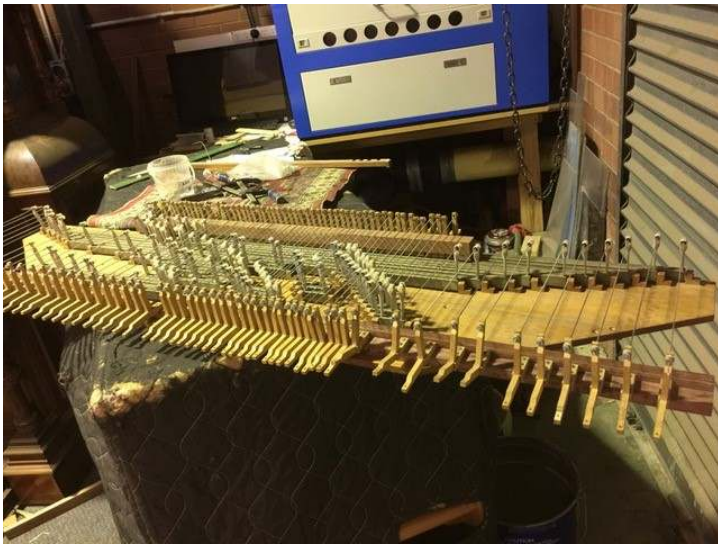
Roller board for the Great division being prepared for installation. It is mounted "upside down" over the top of the Swell roller board.
