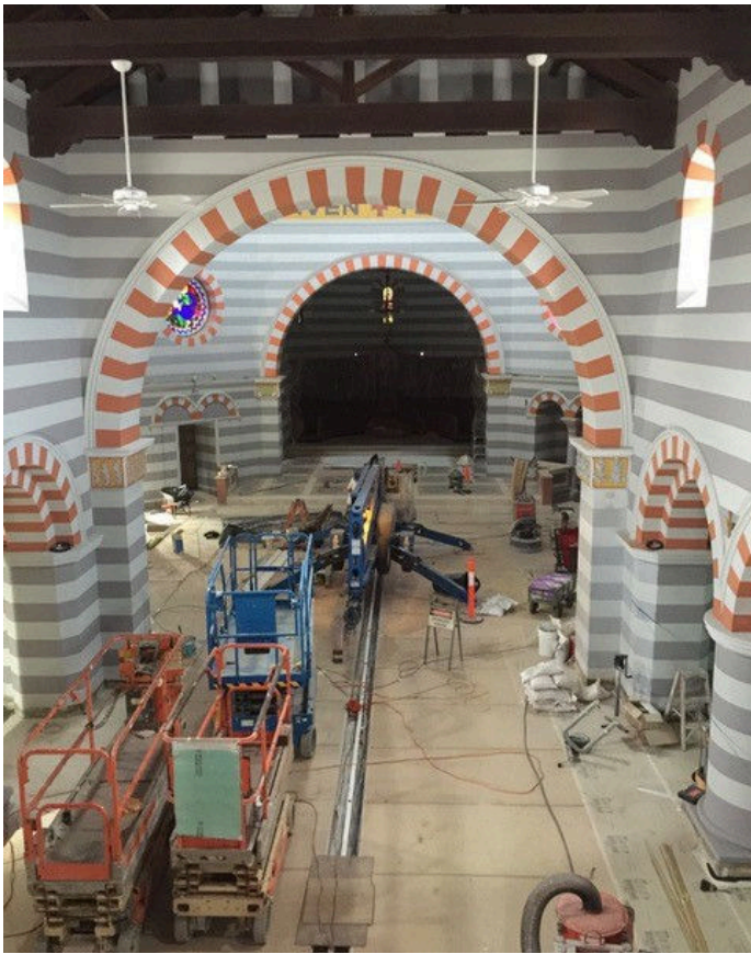
View of the nave from the West End gallery during construction
